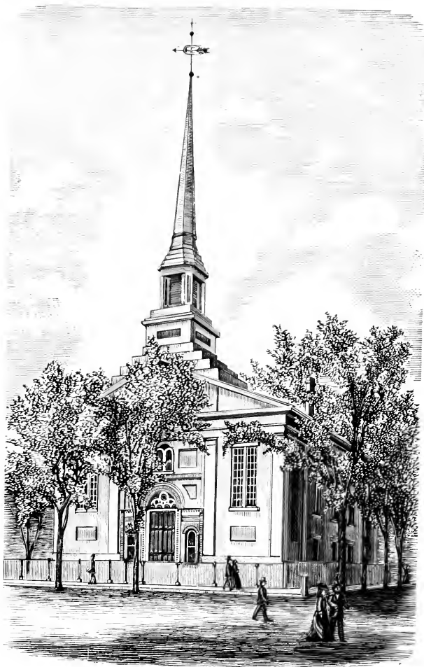
JOHN STREET CONGREGATIONAL CHURCH.
